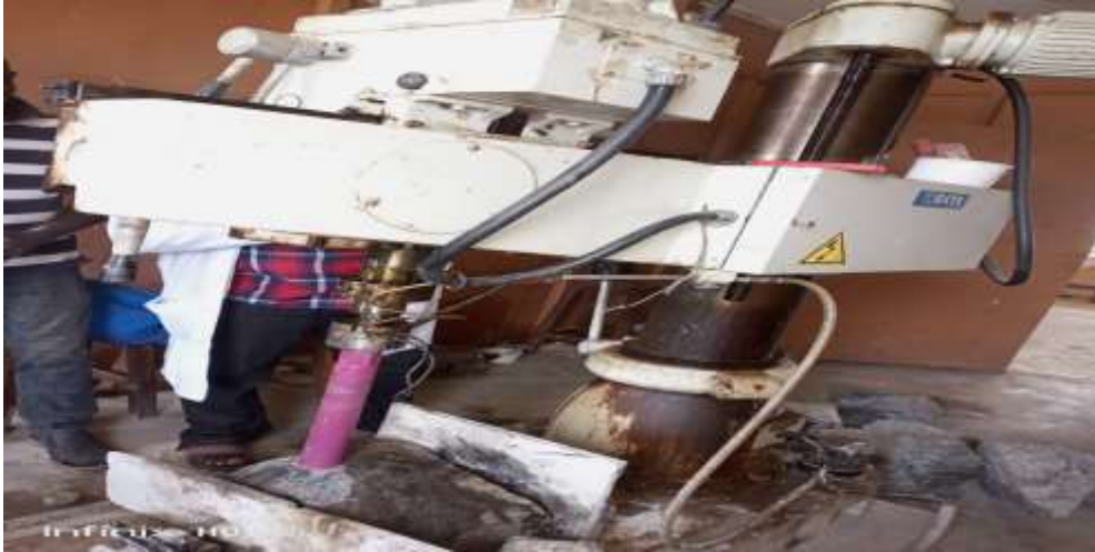
Figure 1: Pillar Coring Machine in Operation
