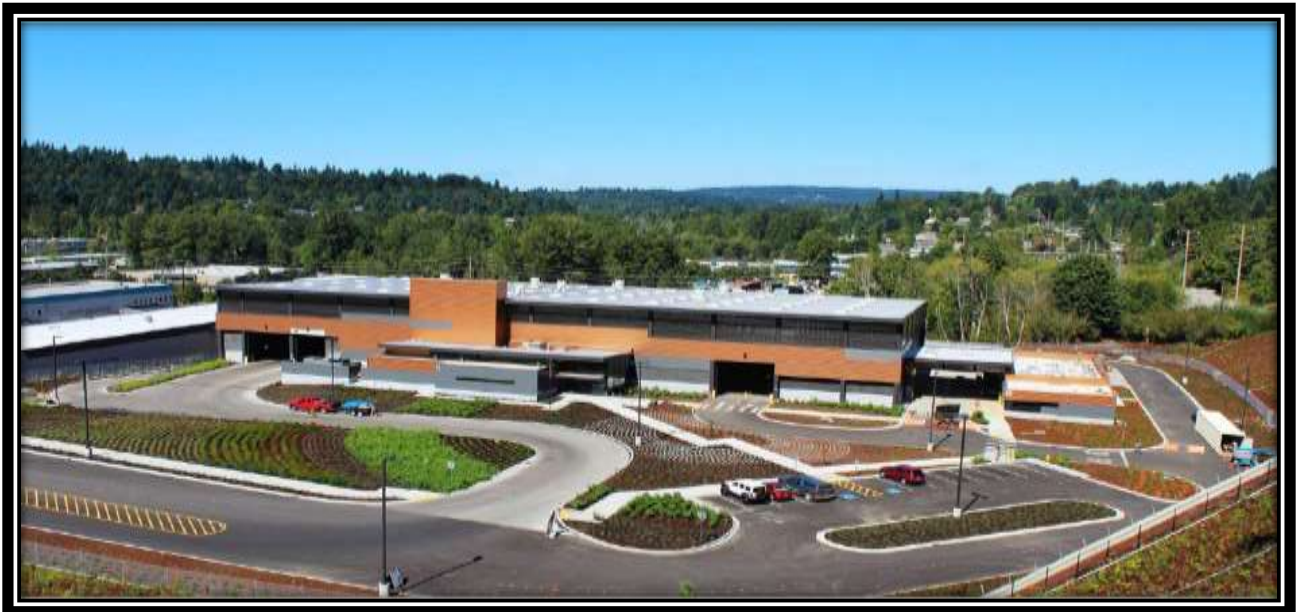
Plate 1: Solid waste Transfer Station Example Source: (Chin, 2018)
