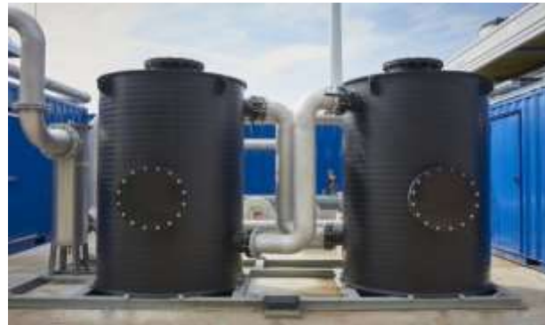
Figure 11: Biogas Scrubbers desulfurization
