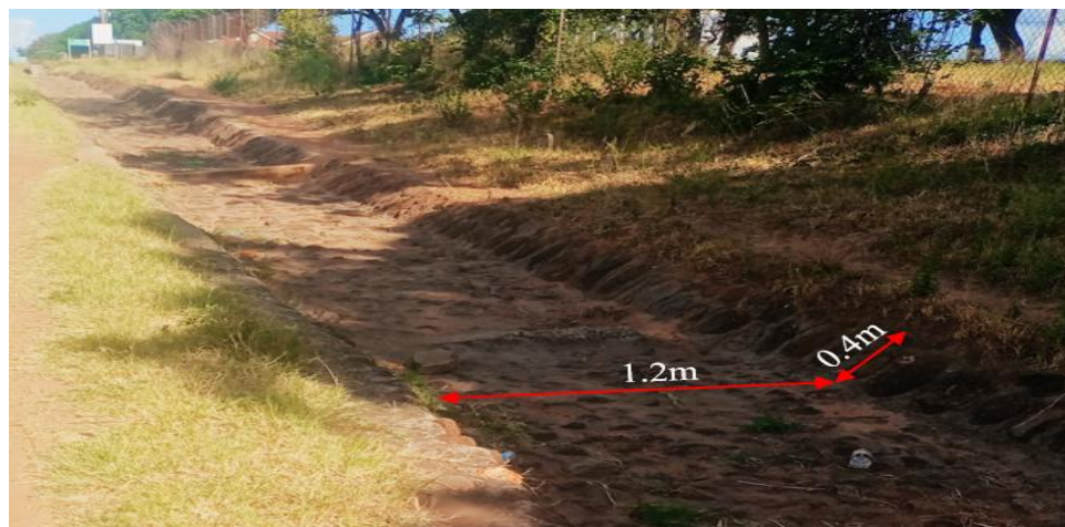
Figure 12: Size estimation of the existing drain on the side of the road adjacent to the gully.
