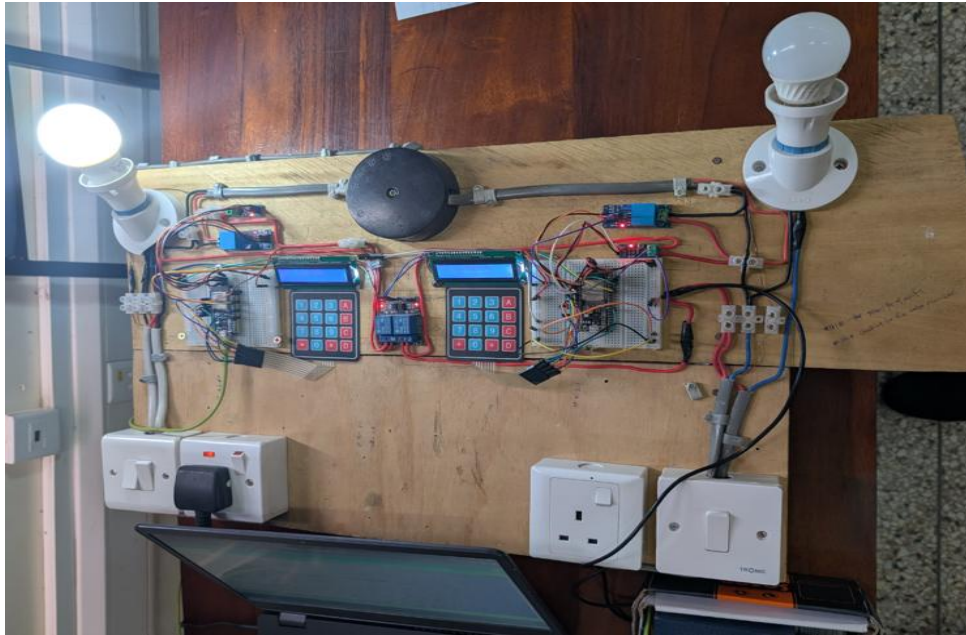
Fig. 3: Functional energy-sharing system hardware prototype
