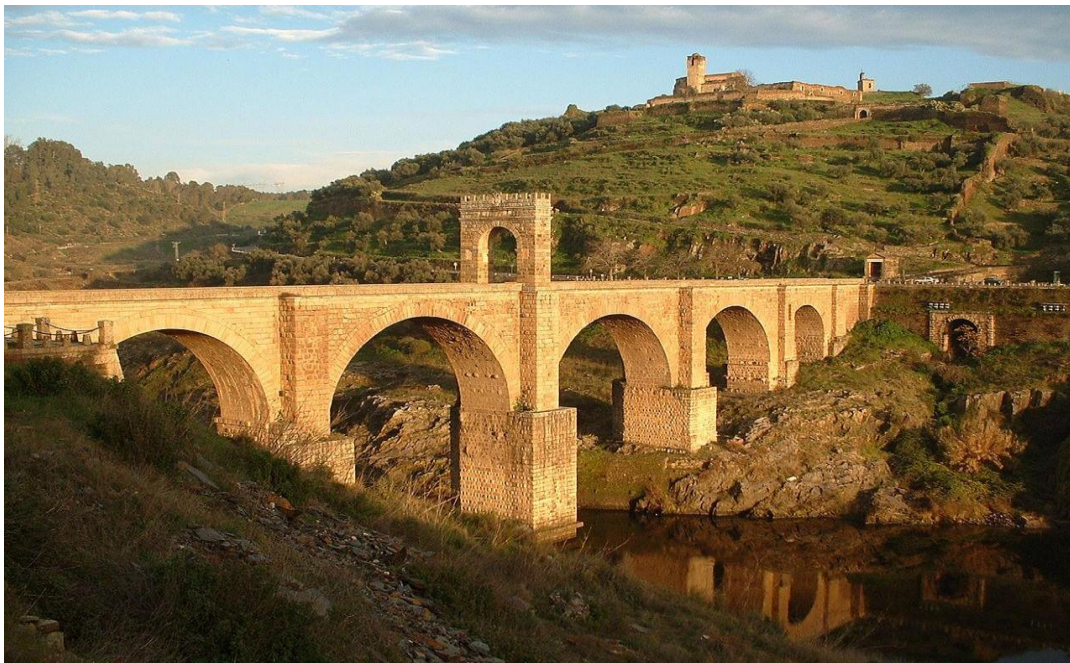
Fig. 6: Roman stone arch bridge built over the Tagus River at Alcántara , Spain between 104 and 106.AD, Span: 194m
