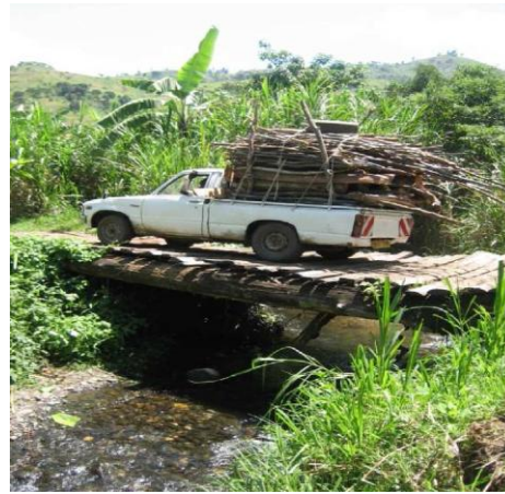
Fig. 2: Timber Log bridges with Limited Span & Strength
