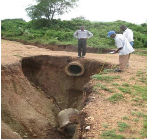
Fig. 1: Eroded Culvert
