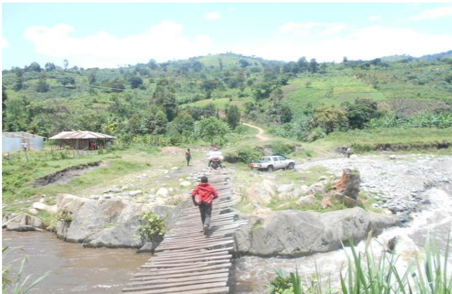
Fig. 3: Timber Bridge at Kyoho, Rwimi River
